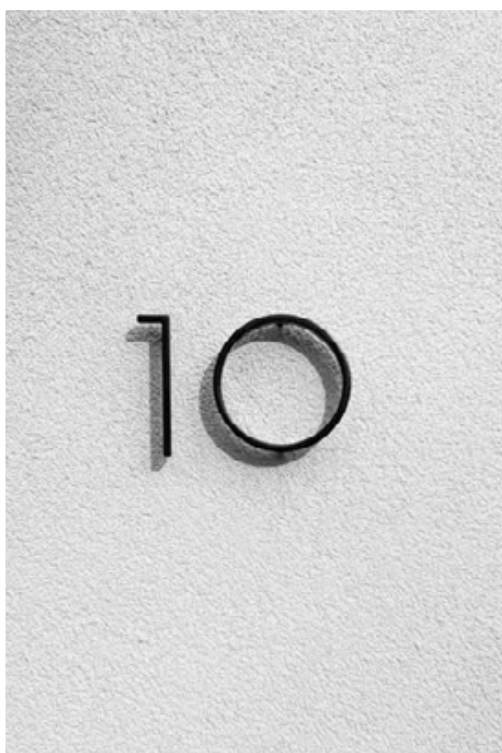
TENANCY SIGNAGE FIXED METAL LETTERING
